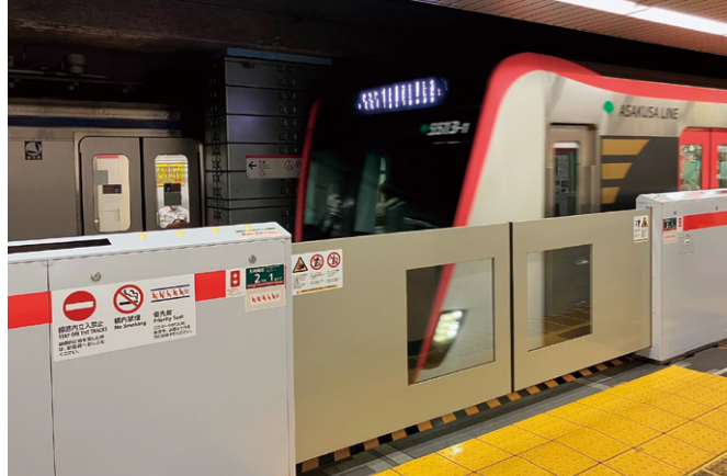
Platform Screen Doors Preventing Accidents
