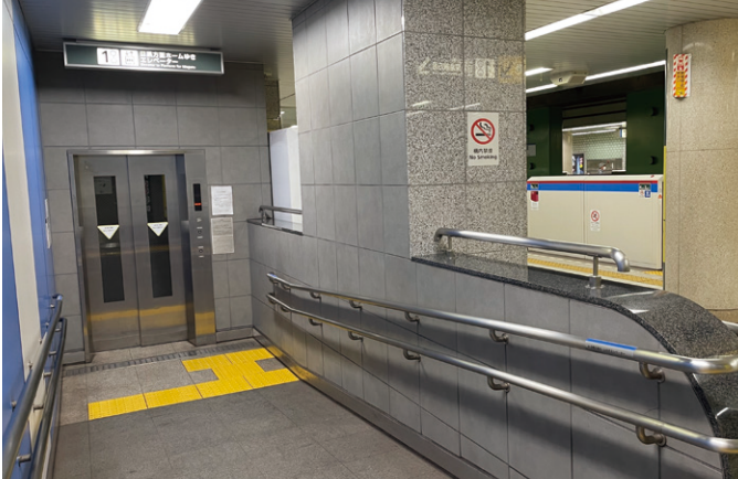
Stairs Eliminated by Installing Elevators
